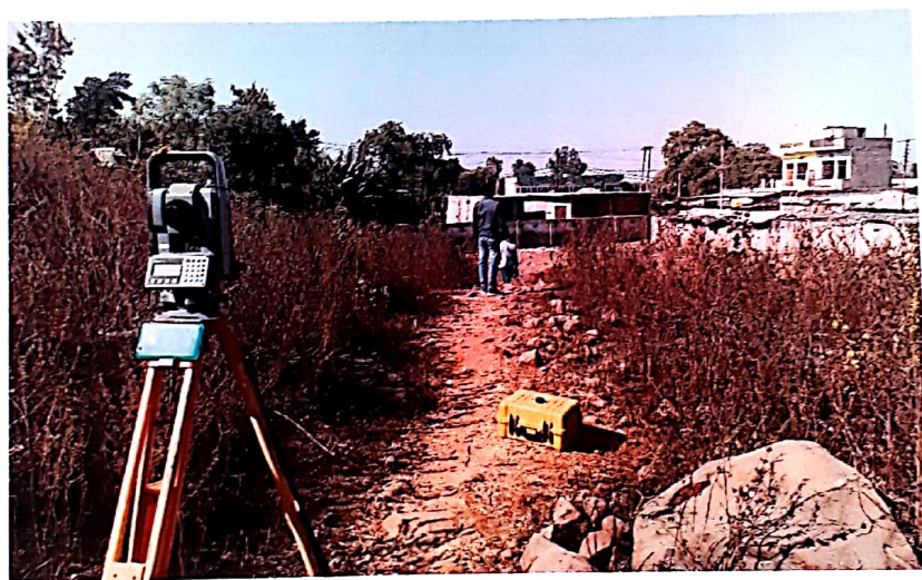
Figure : Topography survey at the site
